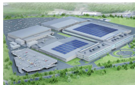
Miyagi No.2 development bldg. (Began operation in Nov. 2018)
